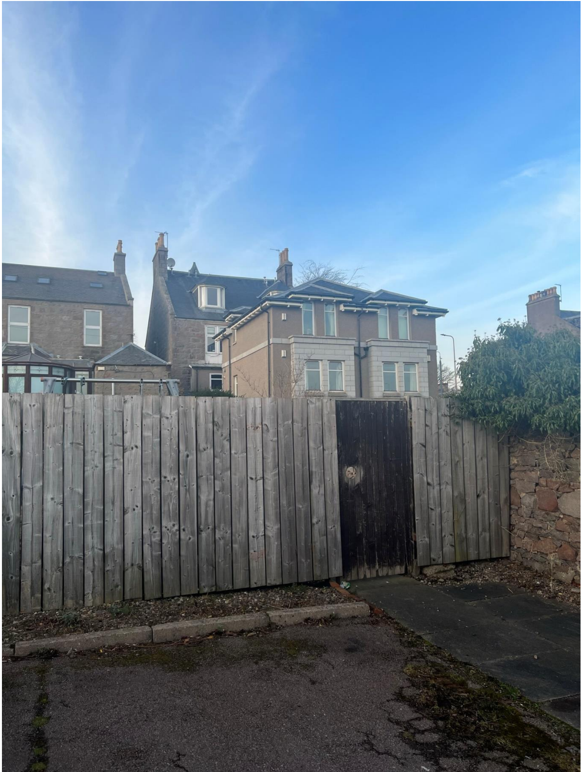
Rear of 449 Great Western Road and 447 Great Western Road as seen from the lane
