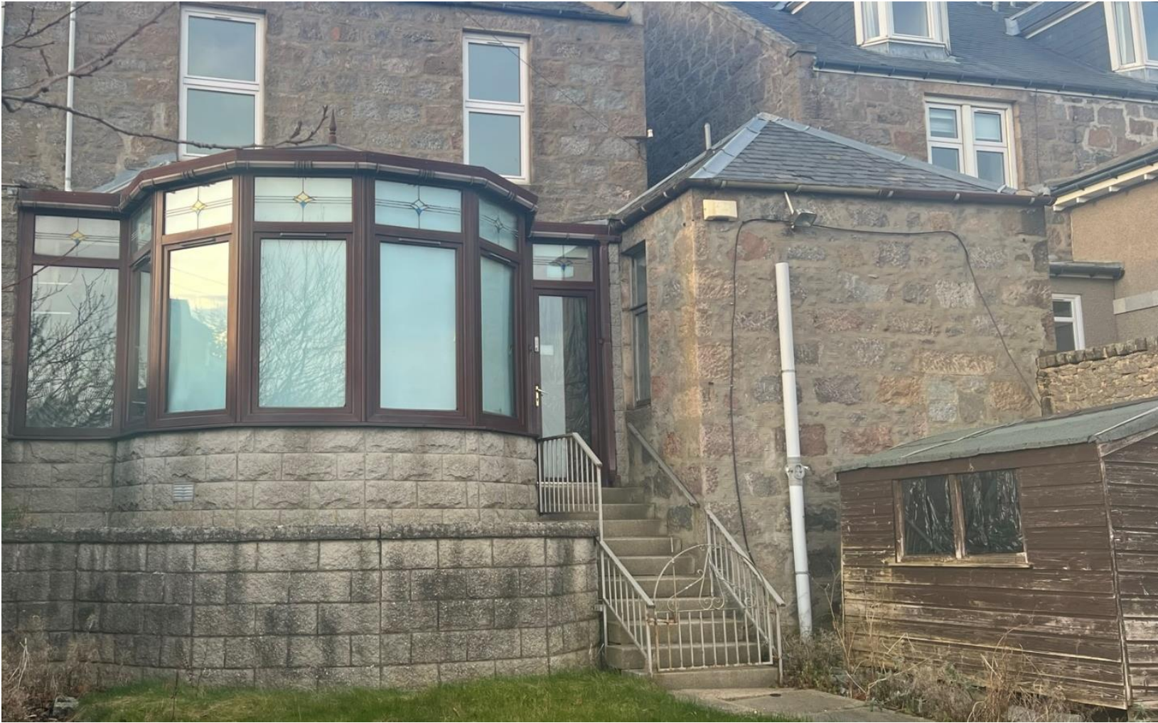
Existing conservatory to rear of 449 Great Western Road and extensions to 447 Great Wester Road as seen from the garden
